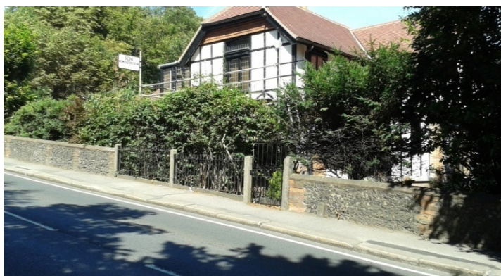
Railings replacing flint walls, St Peters Hill
