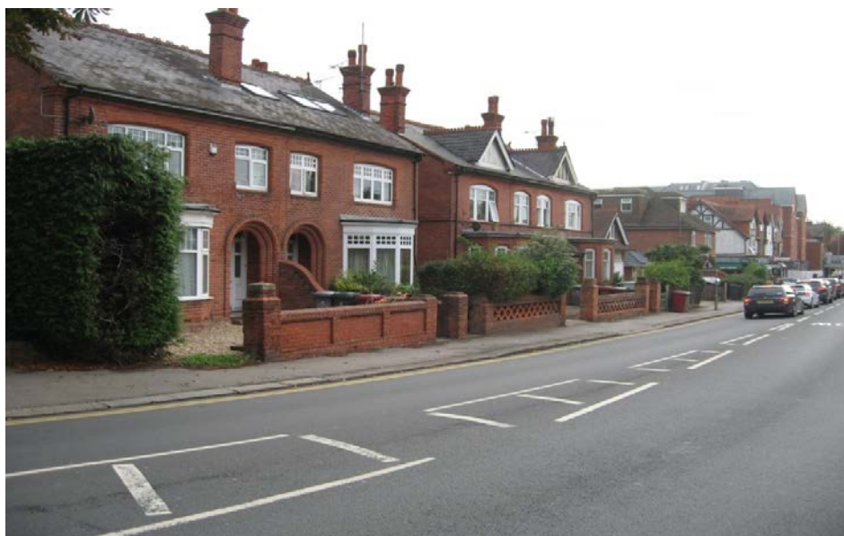
The front gardens and garden walls of these four substantial semi-detached houses in Church Road are under pressure. There is a potential risk to the remaining garden walls which are characteristic of the period in Reading.
